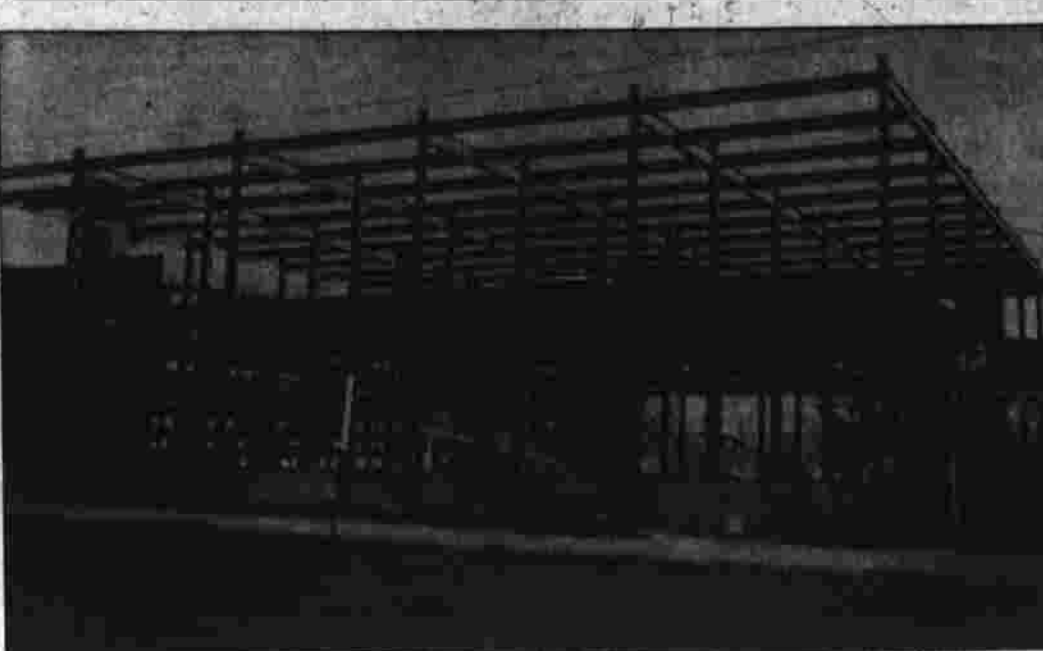
This seemingly ordinary steel structure now going up on E. Center St., next to Manchester's Southern New England Telephone Co. office, will house Connecticut's first electronic telephone system equipment. The new SNETCO building, located on property purchased in 1961, will have approximately an 80-foot frontage and 200-foot depth and provide a new dialing system for telephone users. This new electronic central office stems from 10 years of Bell system research and development, costing more than $100 million, and will be one of many such installations placed throughout the nation in future years, according to Lloyd Hobron, SNETCO manager in Manchester.
